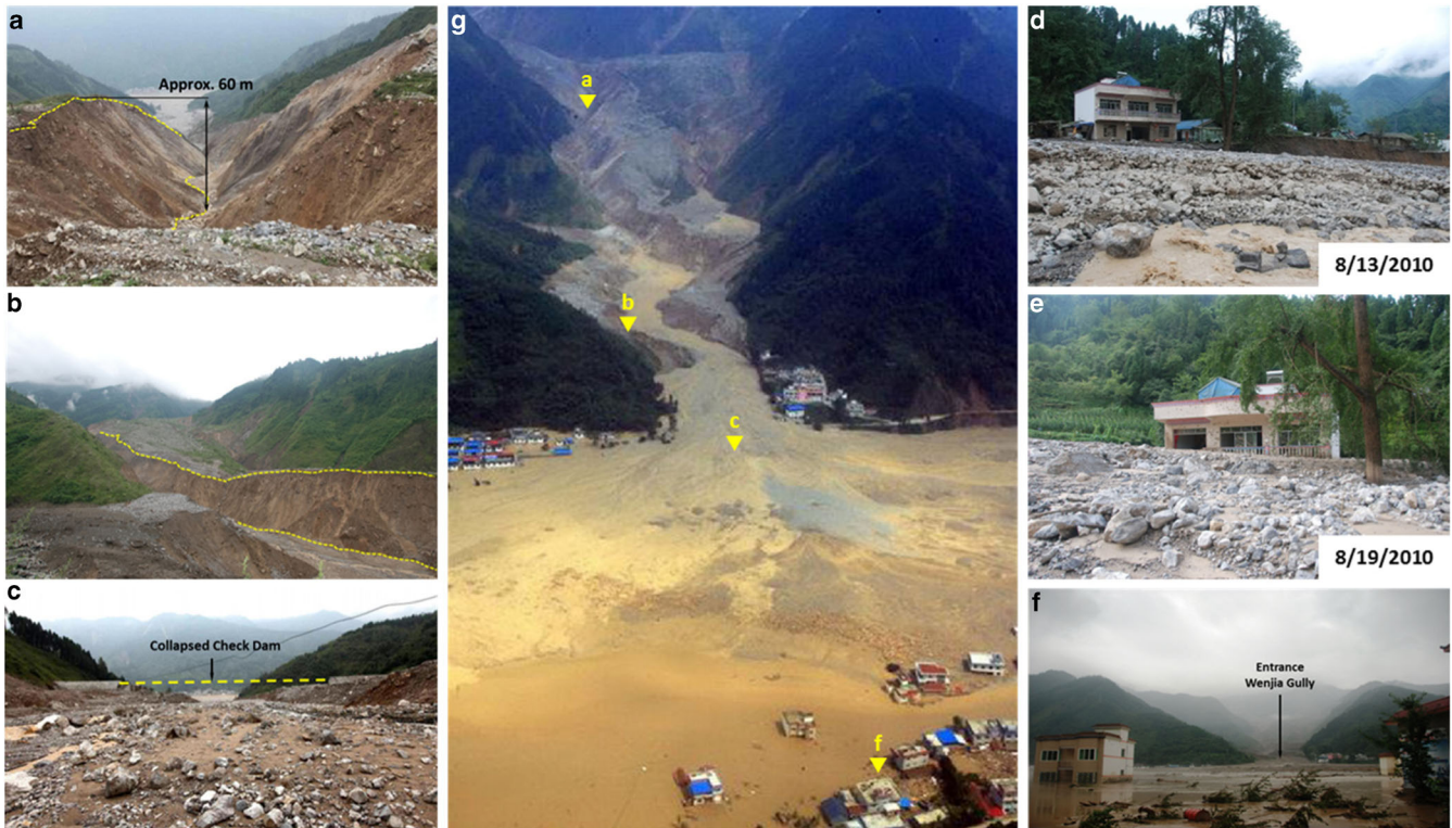
Fig. 3 The devastating debris flow occurred on August 13, 2010. a Deep incision due to channelized erosion on the 1300 m Platform. b Widened debris flow channel near the outlet of the gully. c Failure of the last check dam (after Tang et al. 2012). d A buried house in Qingping Village (August 13, 2010). e Increase in the thickness of the deposit after a subsequent debris flow (August 19, 2010). f Submerged area near the outlet of the gully. g Aerial image of the debris flow with approximated locations of the images presented herein
