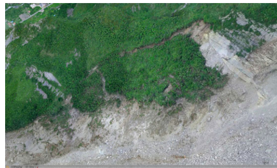
图 19 西侧变形体全景(无人机航拍高清三维模型影像) Fig.19 The high resolution 3D image showing the whole west unstable rock mass
