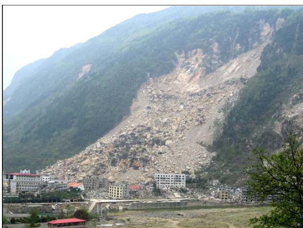
Fig. 10 Overview of the Beichuan New Middle School landslide
